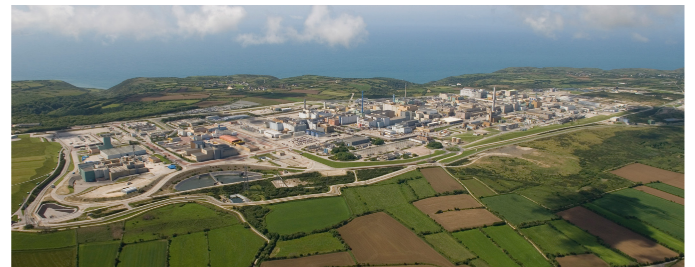
ORANO La Hague, France: over 600 remote manipulators installed.
